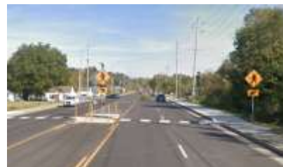
A mid-block crossing was recently installed on Hwy 72 to improve safety for crossing pedestrians and bicyclists
