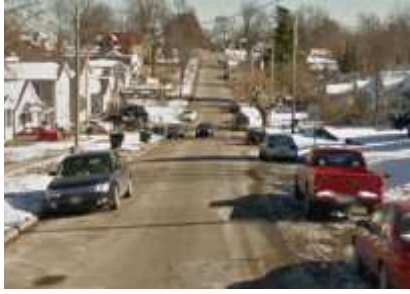
12th Street is 30 feet wide. With on-street parking on both sides, only about 14 feet remains for driving.
