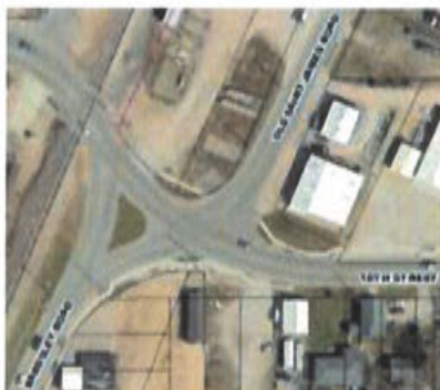
Intersection of 18th Street, Bardsley Rd, and Old Saint James Rd
