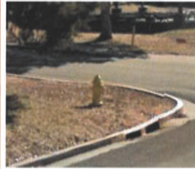
Fire hydrants provide needed water to fight fires and allow water lines to be flushed to keep the water clean. They can also be tested to check the water pressure and water flow in the area.
